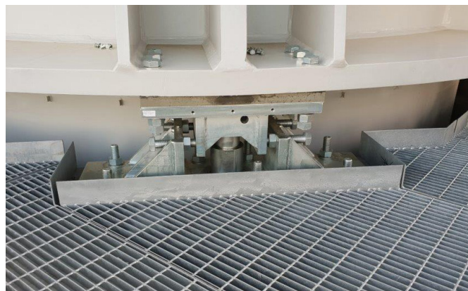
The PR 6201 load cells can accurately weigh loads of up to 12 tonnes.
