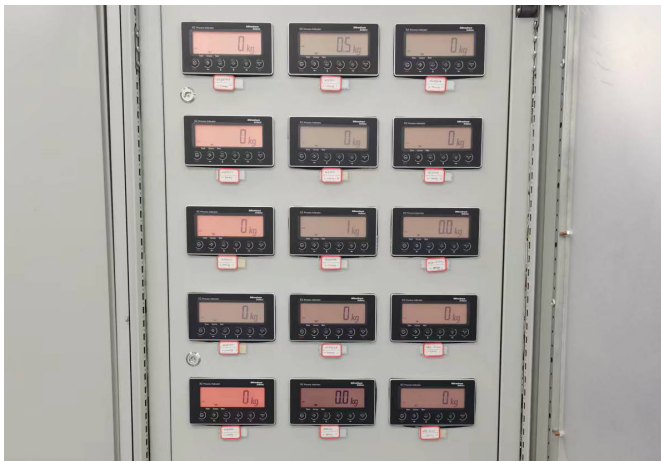
The process indicator X2 in the cabinet reliably shows the weighing results.
